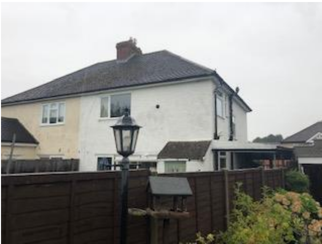
Site photo of rear of No. 28 (host dwelling)
